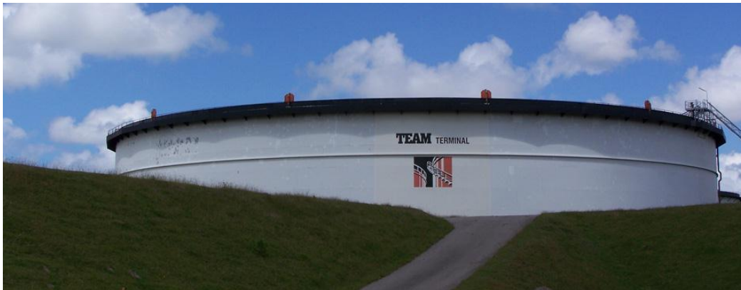
Figure 4. Team Terminal storage facility, Rotterdam
