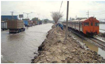
Inundated railway track and road
